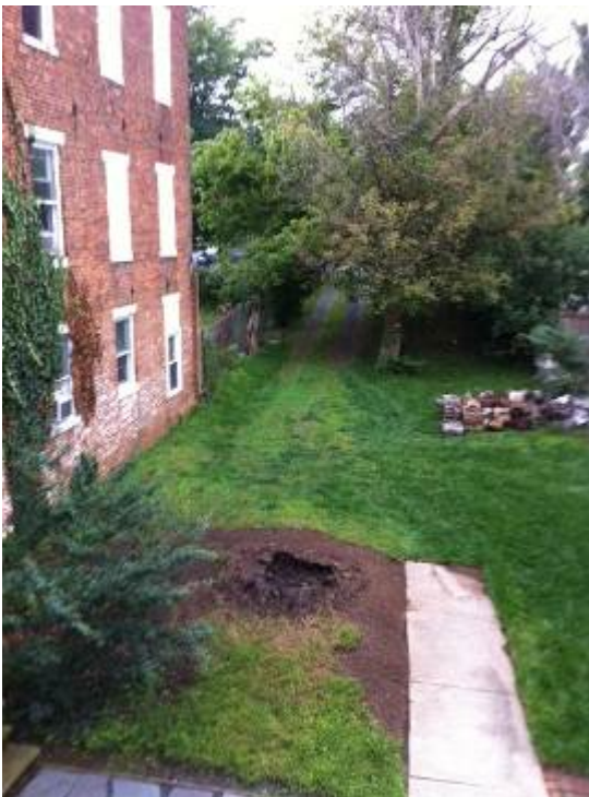
Rear Entrance For Parking
