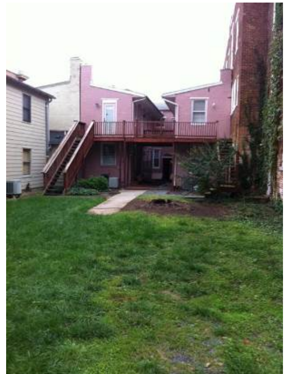
Rear Entrance For Parking
