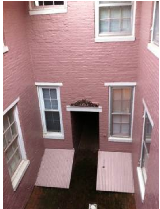
Rear Entrance For Parking
