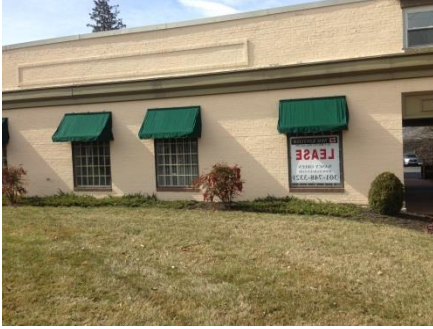
Office Outside View
