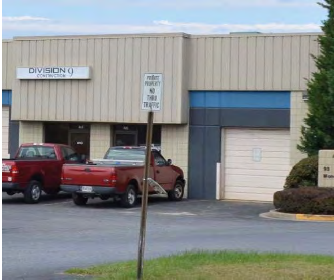
Front View With Drive In Door
