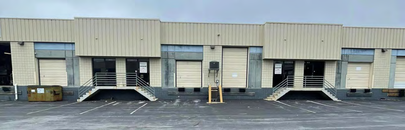
PEBC Suites B10, B11, B12, & B13 Exterior View – With AC, Dock Doors & Restroom
