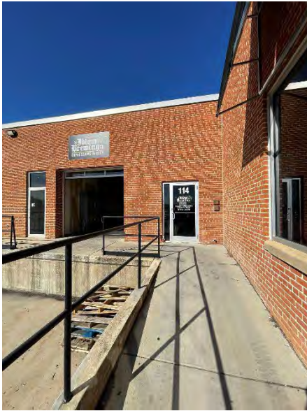
View of Dock Door
