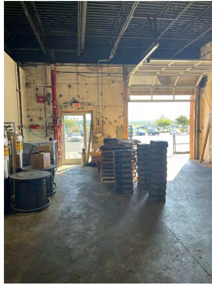
Inside View of Dock Door
