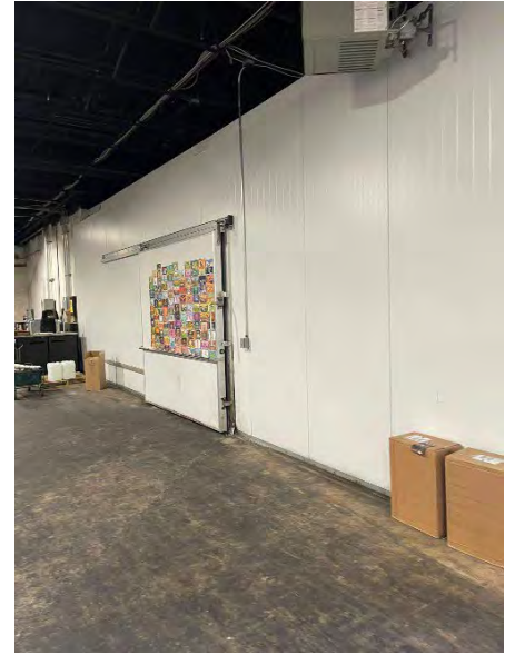
Inside View of Cooler Room
