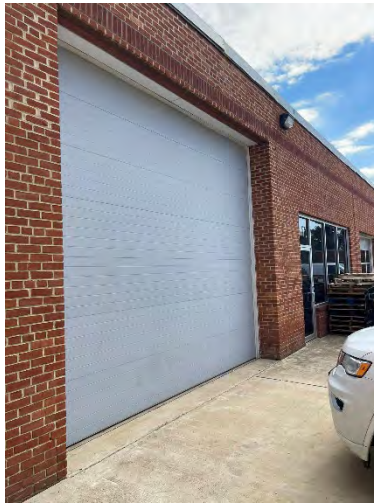
View of Drive-In Door
