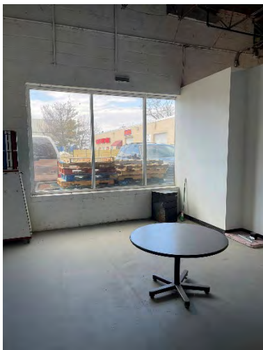
Inside Entrance Office
