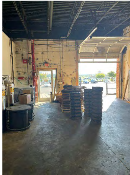
Inside View of Dock Door
