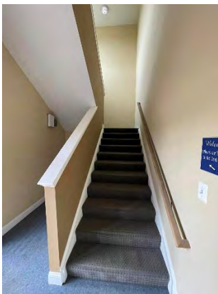
One of Two Stairwells
