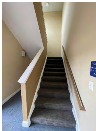
One of Two Stairwells
