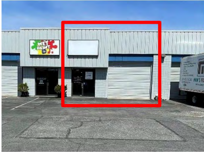
Front View with Drive In Door
